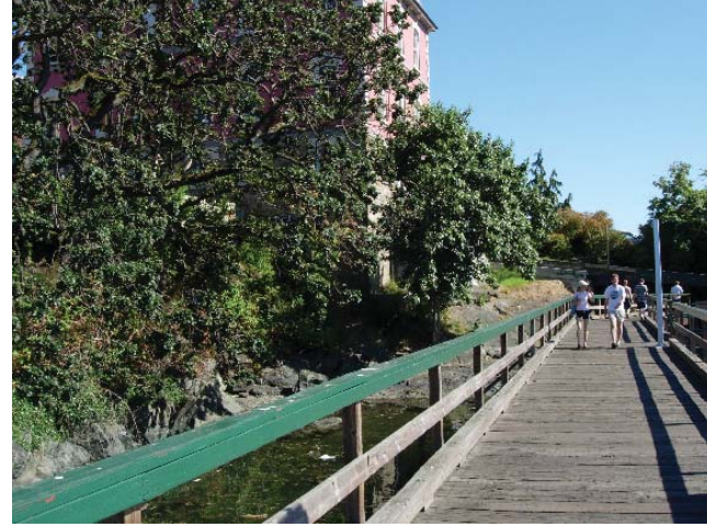
Existing Boardwalk/Bridge :Downtown/Old town Victoria
