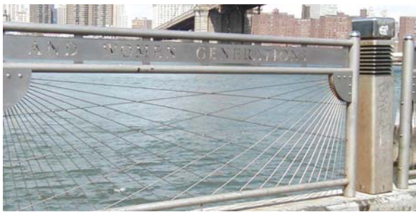
Bridge Example Railing:New York
