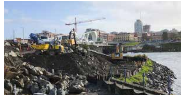
Construction continues at Songhees Park
