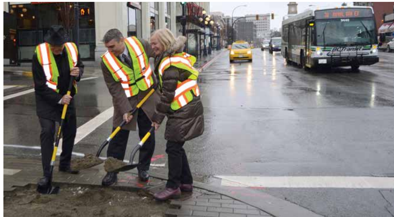
Work begins for new transit lanes
