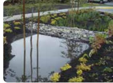
**Sizing:** Must treat at least 25 m<sup>2</sup> (270 sq. ft.) of roof or other hard surfaces
