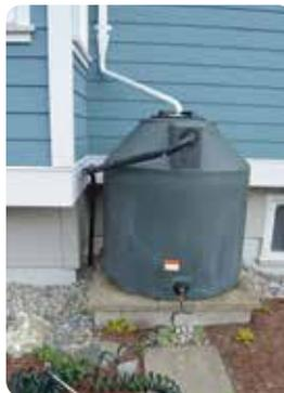
**Sizing:** Minimum 1,200 litres, must treat 25 m<sup>2</sup> (270 sq. ft.) of roof
