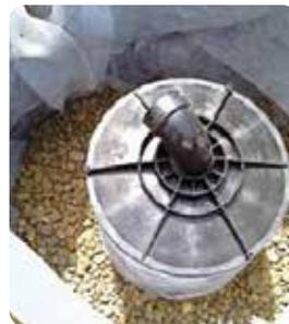
**Sizing:** Must treat at least 25 m<sup>2</sup> (270 sq. ft.) of roof or other hard surfaces
