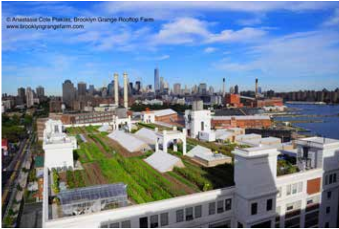
Brooklyn Grange Farms in New York City operates two rooftop vegetable farms made of raised beds on an intensive green roof totalling 1.4 hectares.
