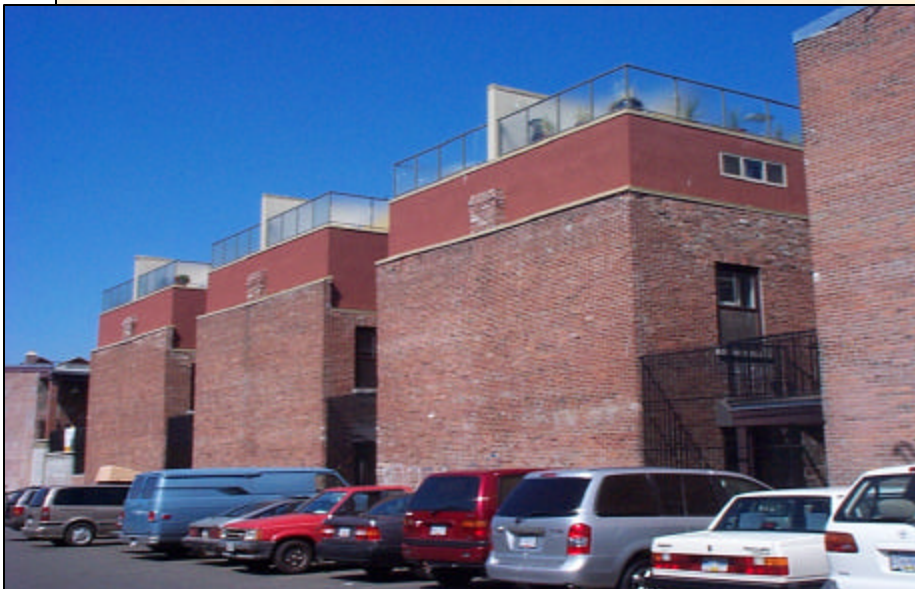
Completed Live work townhouses
