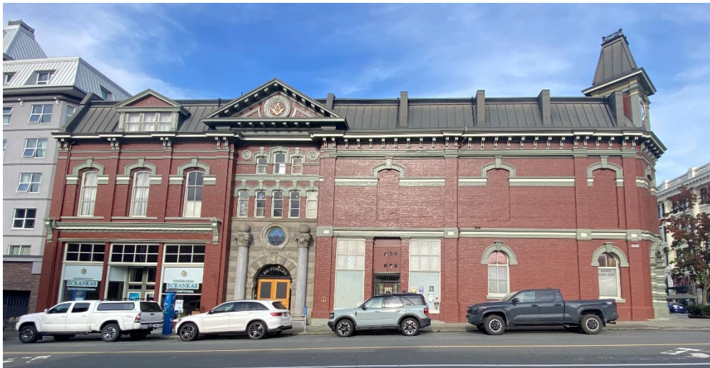
Fisgard Street (South) façade
