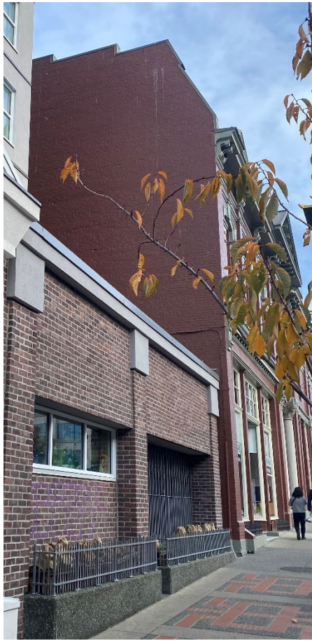
Side (West) façade
