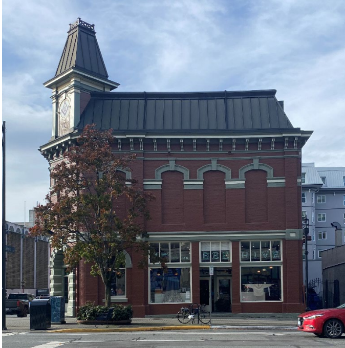
Douglas Street (East) façade
