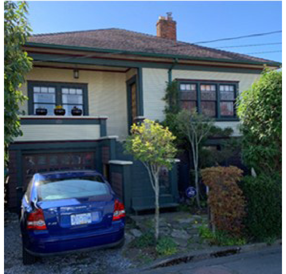
53 Lewis Street, built 1929.
