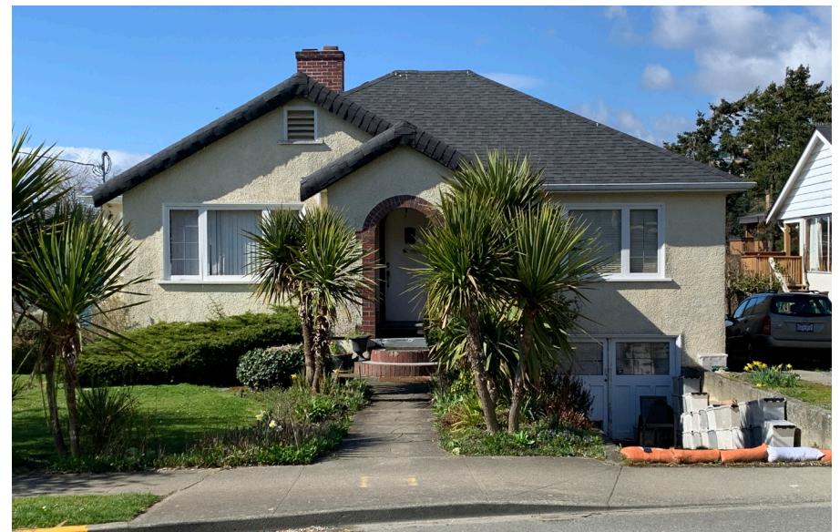
206 Robert Street, c. 1945, Constructed by A. Petek for Mr. George Goy. Rolled eaves and bricks embedded in plaster are references to the English Cottage Style.
