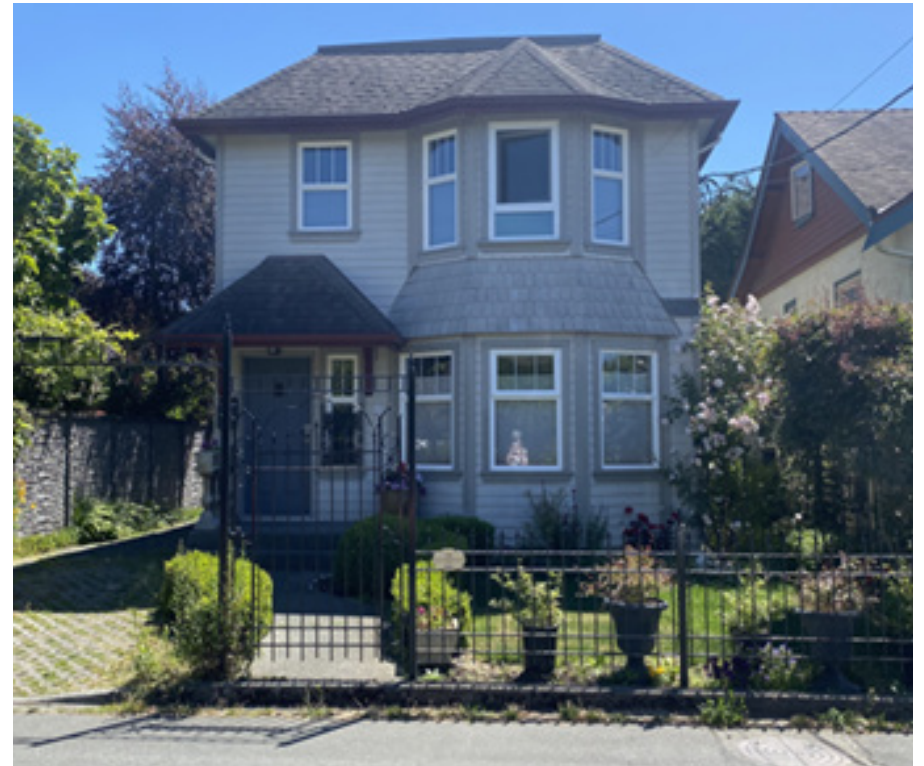
Lewis Street was built in the 1990s and fits well within the street. Its form, scale and massing are all sympathetic to the context, and the details and features such as the angled bay and covered front entry are modern interpretations of common features of the historic homes on the street.
