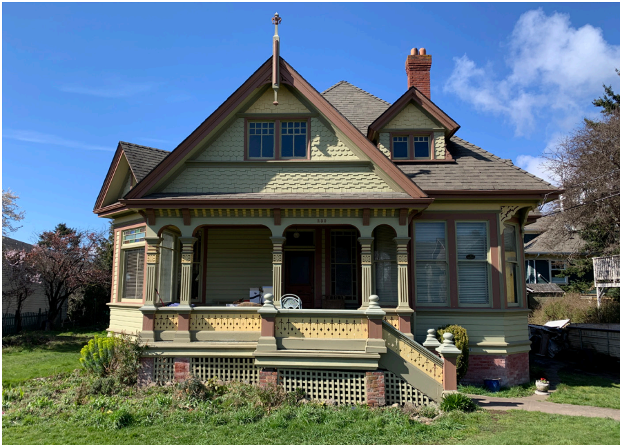
230 Robert Street, c. 1899-1900, Architect: Thomas Hooper.
