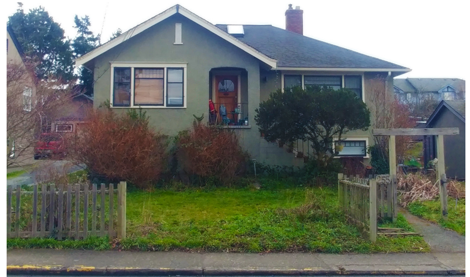
255 Robert Street, c. 1940, Constructed by N.A. Thomas for Howard Horner, who was a trainman for the Esquimalt and Nanaimo Railroad.
