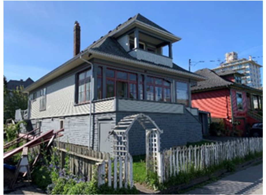
39 Lewis Street, built 1908.
