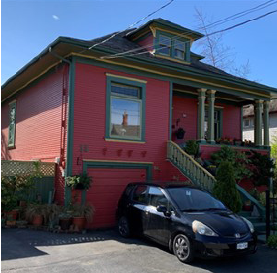
35 Lewis Street, built 1907.
