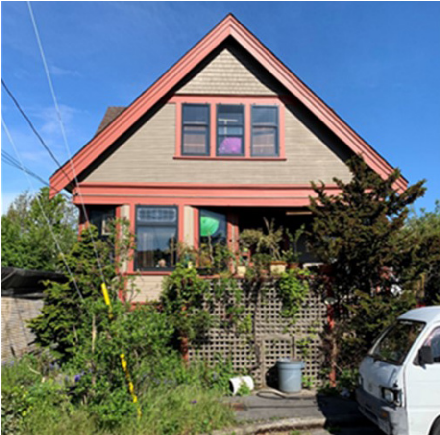
50 Lewis Street, built 1912.
