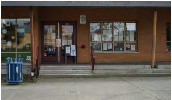
Quadra Village Community Centre
