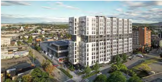
2615-2629 Douglas St. D'Ambrosio Architecture + Urbanism
