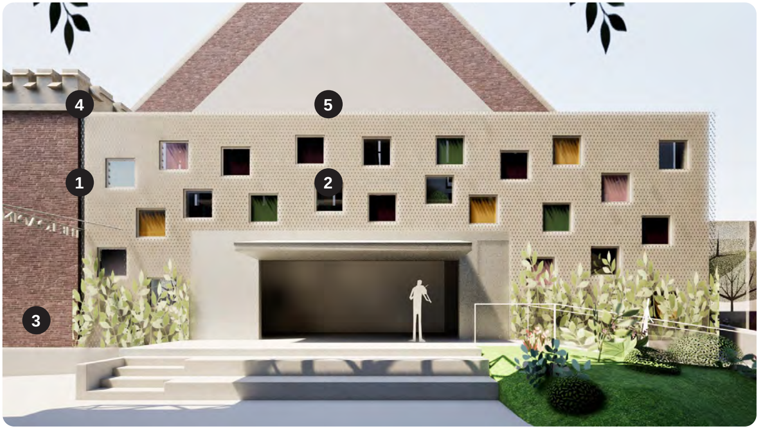
Materiality and detailing to distinguish heritage character. The facade intersections between the East Addition and the First Met Heritage Building are articulated with concrete reveals, and a distinct material palette for the new construction.
