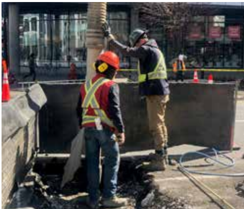
Blanshard Street water main upgrades
