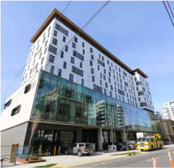
Victoria Fire Department Headquarters
