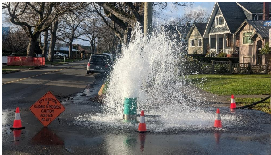
Photograph 4: Watermain Flushing
