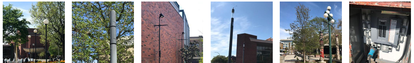
Lighting inventory and electrical box example
