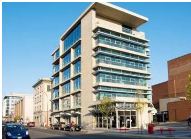
New CRD building, 2006
