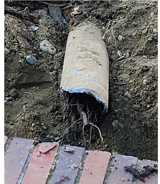
Figure 2: Tree roots in conflict with existing on-site utilities.
