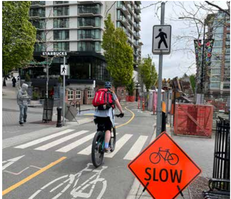
Longer term use of AAA bike lane is re-aligned to ensure it remains open and accessible while providing space for construction
