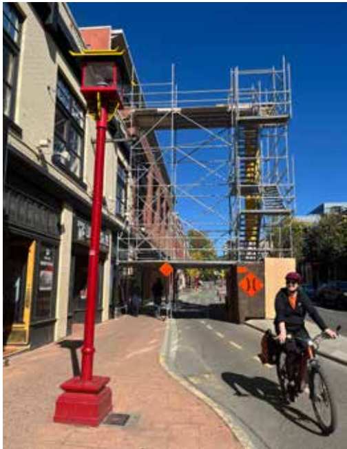
Overhead scaffolding leaves sidewalk and protected bike lane clear and accessible.
