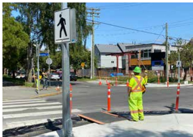
A temporary curb ramp allows access to the crosswalk from the sidewalk
