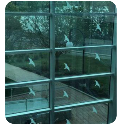
Above: Examples of glass treatments and designs that reduce the likelihood of bird strikes.
