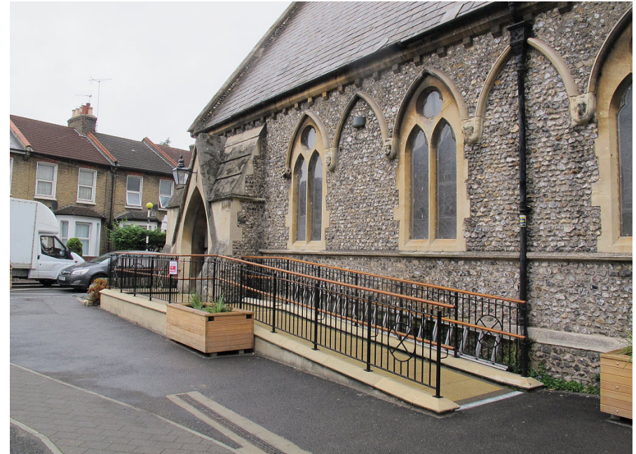
Access ramp and its elements are designed to be integrated into the building and site at a heritage church.
