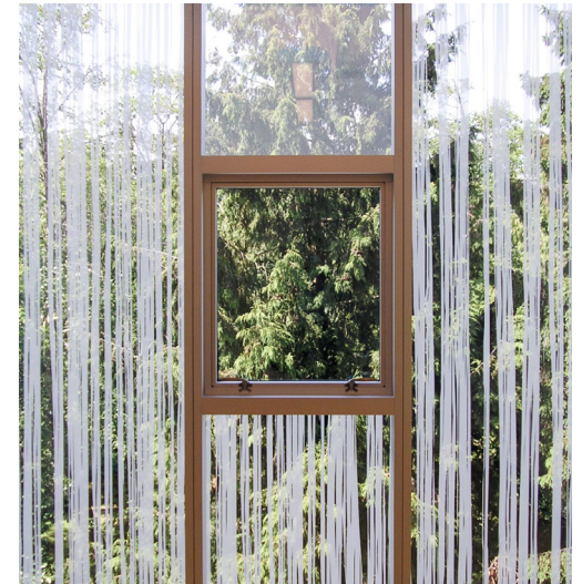
Frit pattern glazing supports bird-friendly design at a research and teaching facility.
