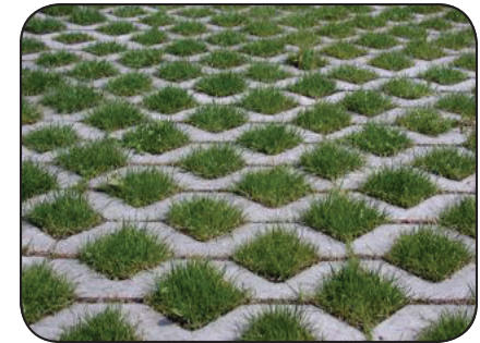
Image 17: 'Permeable Surface Design' Cellular Concrete Pavers in which natural grass can be grown
