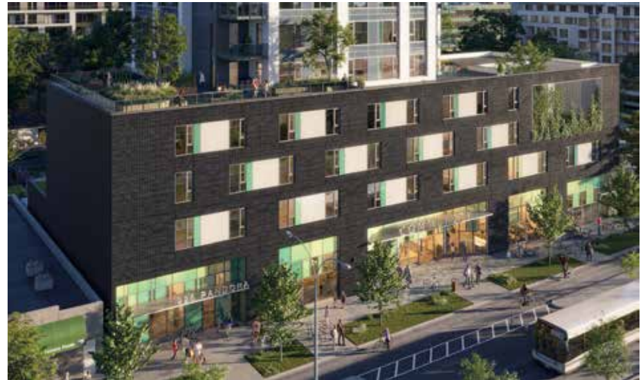
926/930 Pandora delivered in partnership with Capital Region Housing Corporation is under construction and will deliver 158 affordable and 47 supportive housing units
