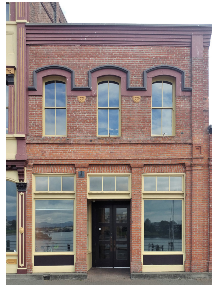
Historic Building – Wharf Street
