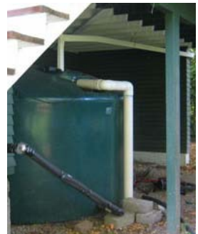
Cistern located under a porch
