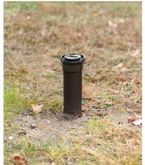
Underground oil tank fill pipe used to refill the tank with oil.
