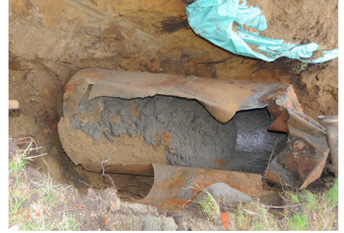
Excavated oil tank.
