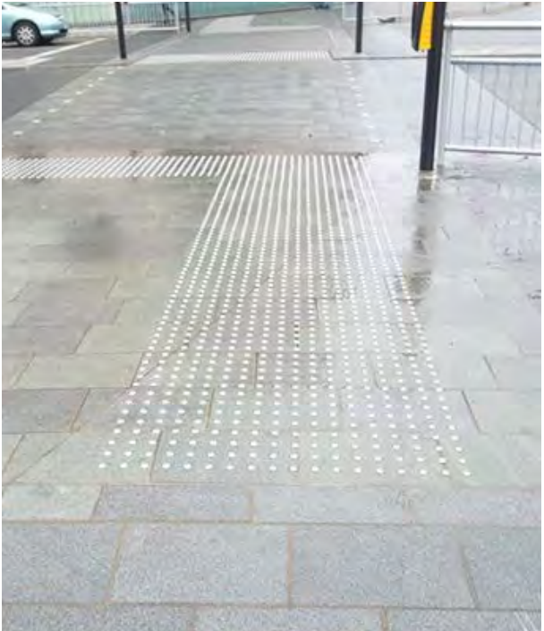
Tactile warning strips combined with perimeter crossing markings provide dedicated crossing zones for the visually impaired.
