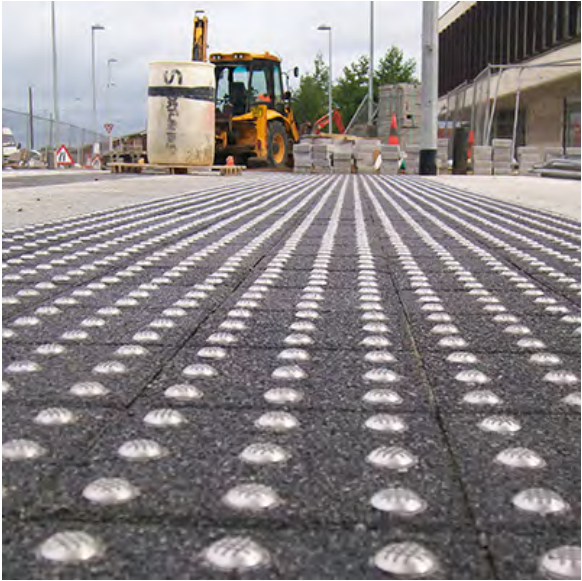
Stainless steel tactile paving studs installed on concrete unit pavers function as warning strips
